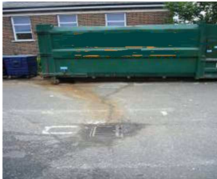
Compactor run-off polluting surface water
