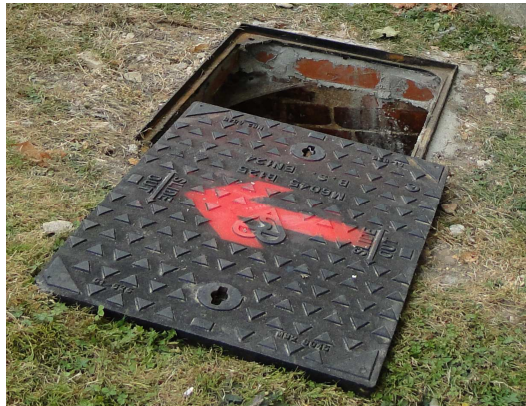
Drain marking – red for foul – on a hospital site.
